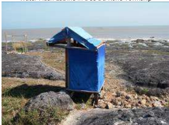
Water Flush Latrine in Dee Du Kone Township
