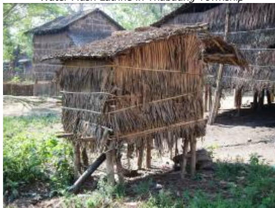
Water Flush Latrine in Thabaung Township
